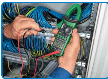
Voltage testing in switchgear cabinet
