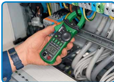
Current measurement in switchgear cabinet
