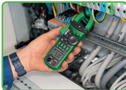
Current measurement in switchgear cabinet
