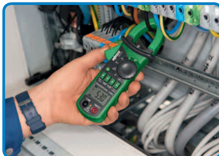
Current measurement in switchgear cabinet
