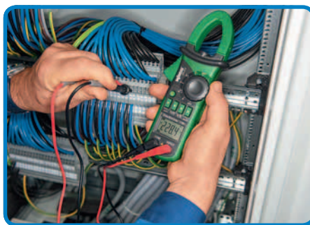
Voltage testing in switchgear cabinet
