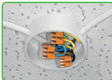
Lighting distribution in ceiling canopy
