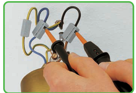
Testing through separate test slot.
