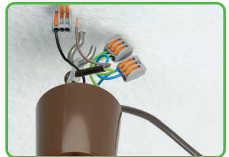
Lighting fixture connected with flexible power feed.
