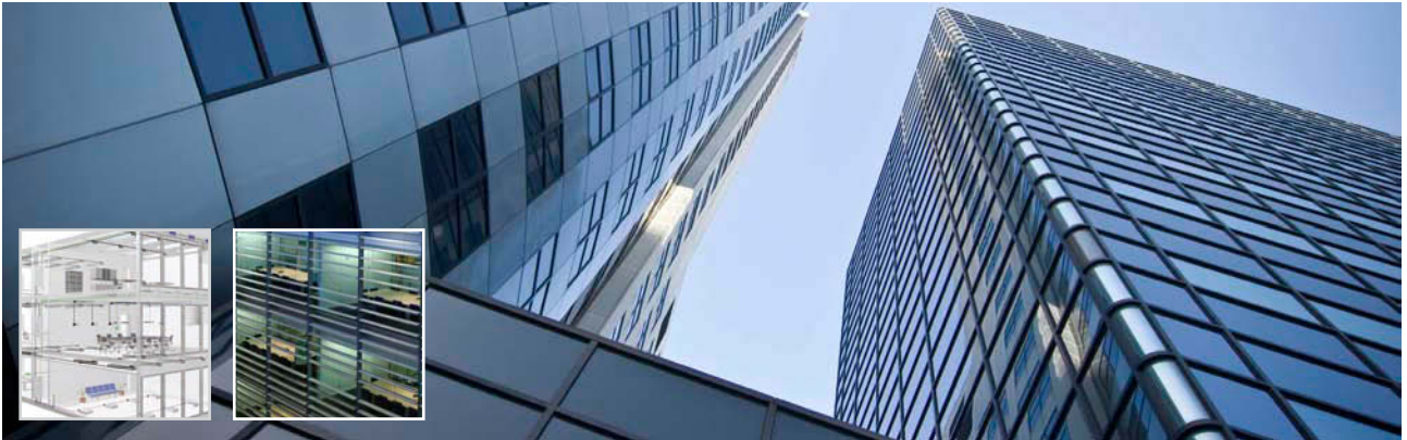
Building installation and automation
