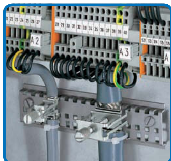
Installation on a specialty slotted carrier rail
