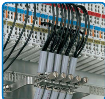
Installation on U-shaped copper busbar
