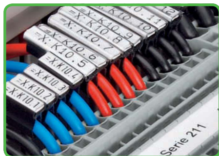
Conductor marking using marking sleeves.
